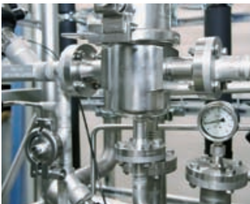
Stainless-steel piping with NEUMO BioConnect flange connections.
